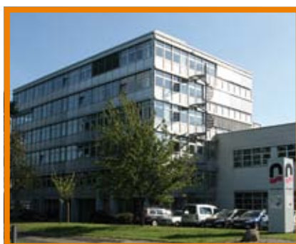
nass magnet: Corporate office in Hanover, Germany
